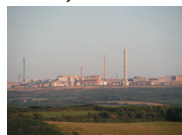
La Hague Reprocessing Plant, France
